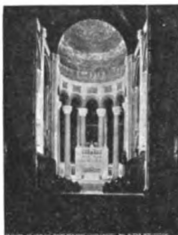
Church Ceiling Diffusers Frink and J-M Linolite
