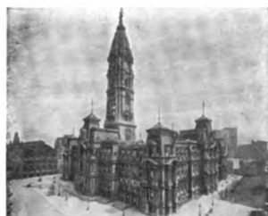
Philadelphia City Hall Roofed With J-M Asbestos Built-Up Roofing
