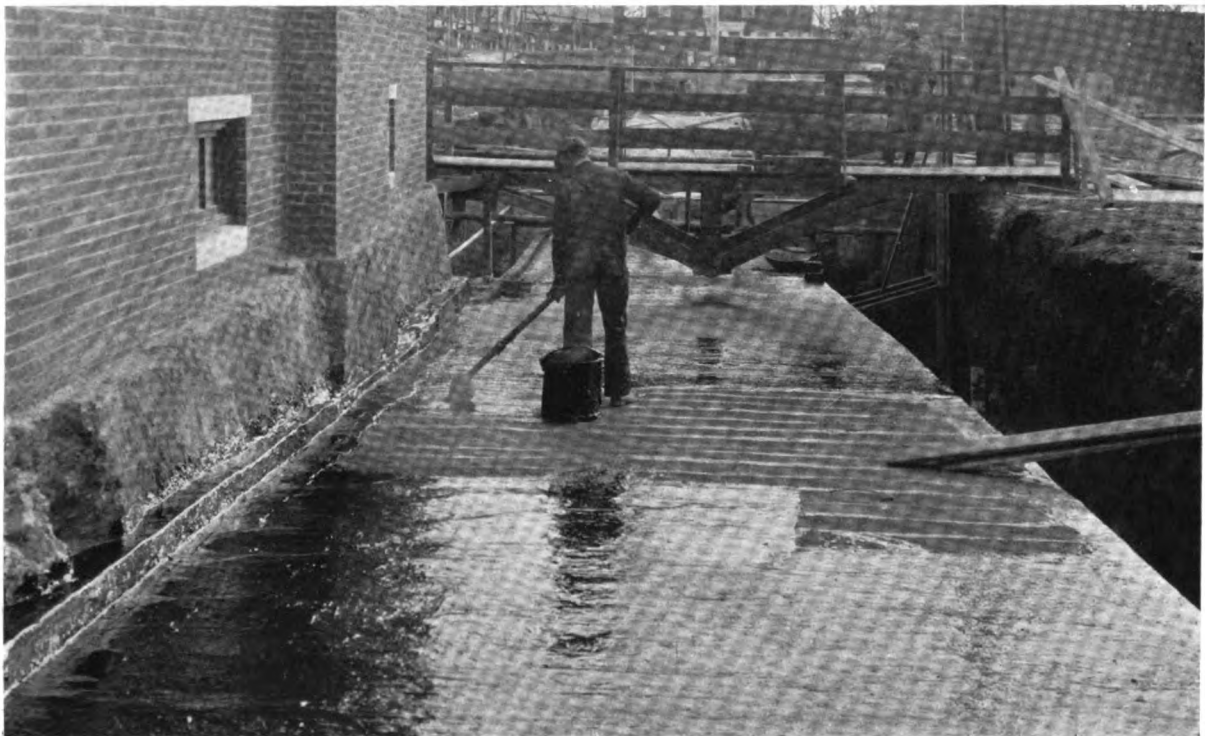
J-M Waterproofing on sidewalk vault, Media County Court House, Media, Pa.
