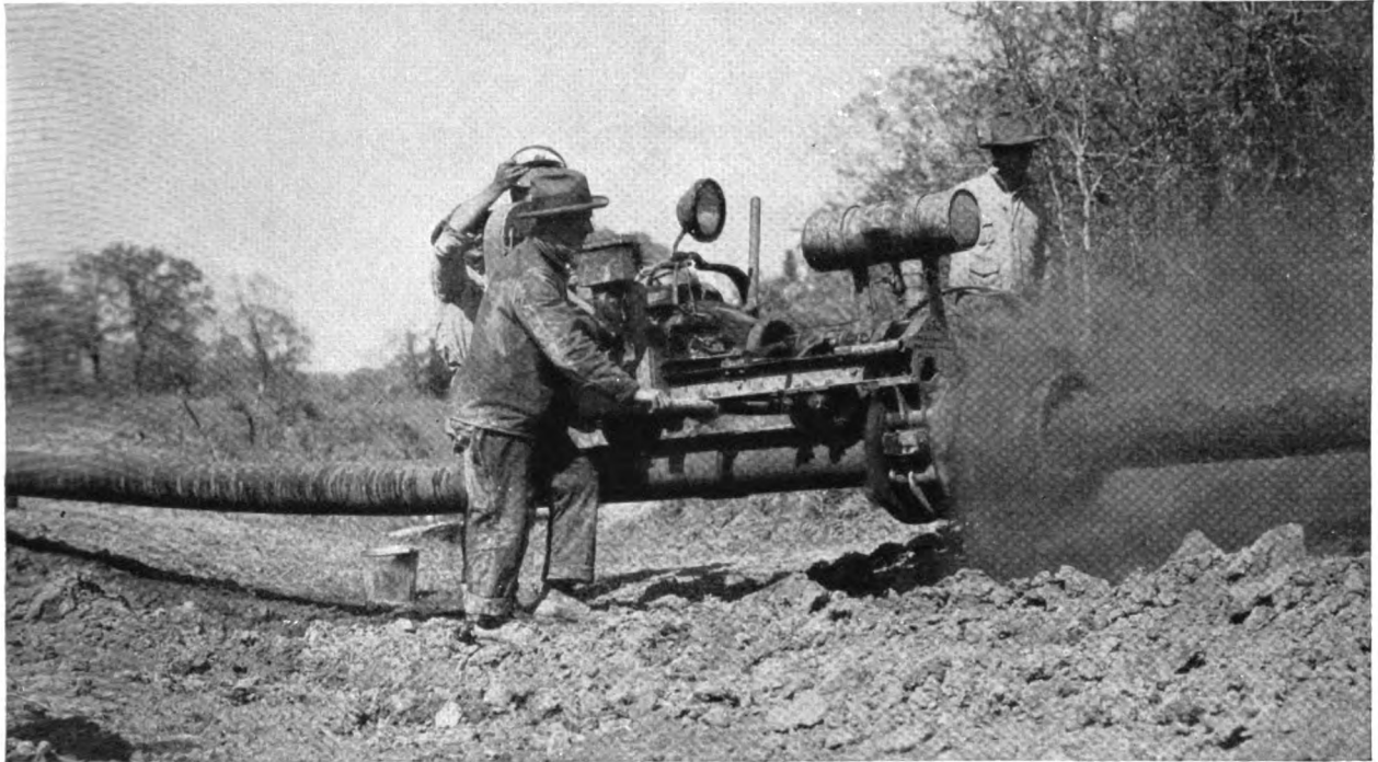
A traveling type cleaning and priming machine in operation—(Photograph through courtesy of the W-K-M Co.)
