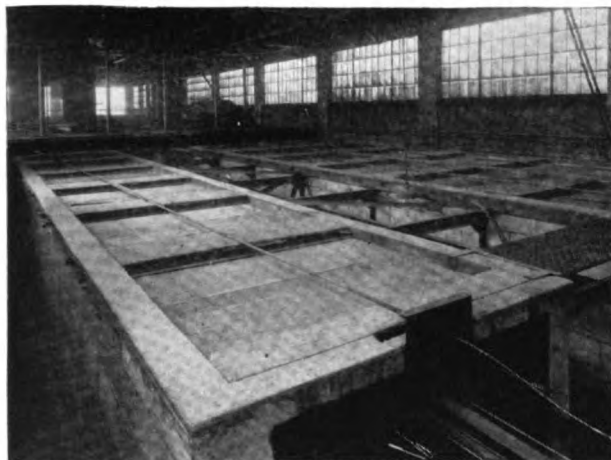
Large japping ovens at the Durand Steel Locker Co., Chicago Heights, Ill., built entirely of Sil-O-Cel C-3 Concrete with 9" thick walls and tops. Size of ovens 9 ft. wide, 22 ft. high, 50 ft. long
