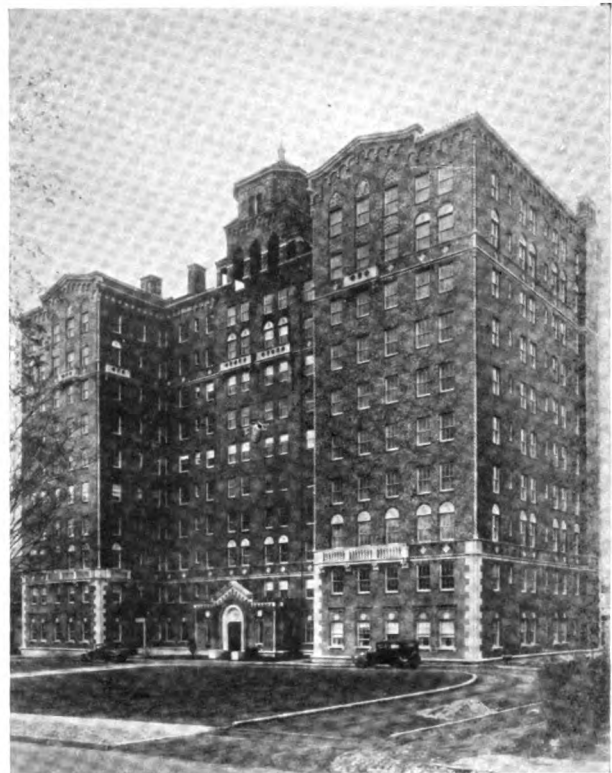
Fig. 4. 75 Prospect Street Apartment, East Orange, New Jersey, 0.6 cu. ft. (6 lb.) Celite per bag cement in 1:3 mix for mortar. Concrete made with 0.3 cu. ft. (3 lb.) Celite per bag cement in 1:2:4 mix. John B. Peterkin New York, Architect; Salmond Scrimshaw Co., Arlington, New Jersey, Owners and Contractors
