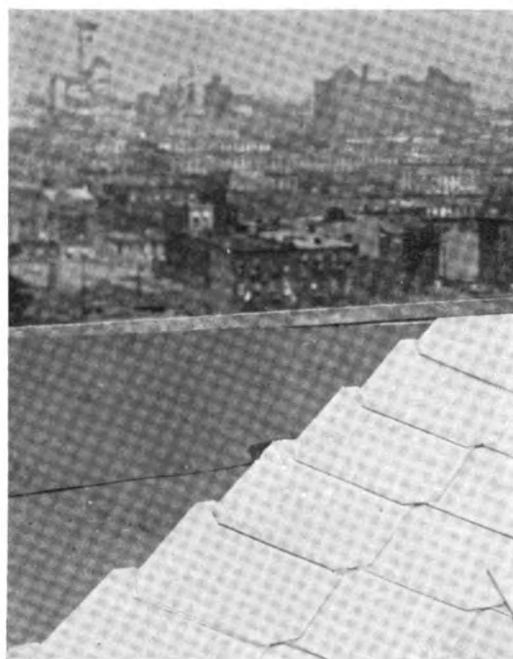
Asbestos Slater's Felt as a liner under Asbestos Shingles
