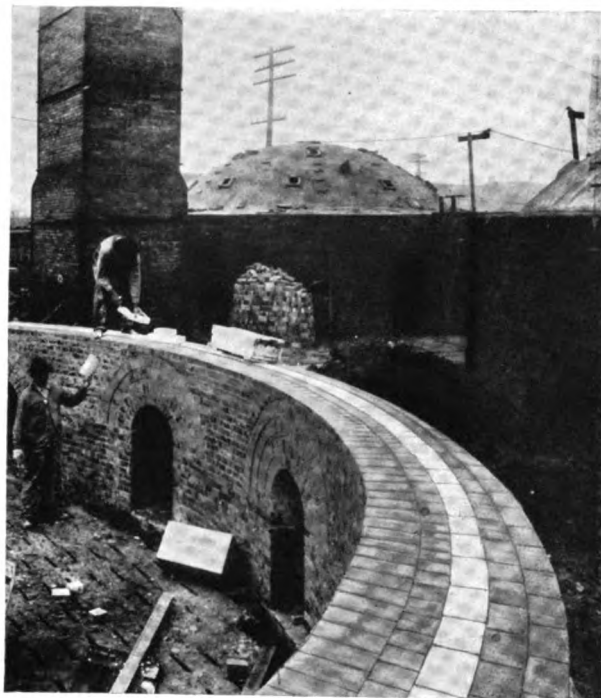
"Core wall" of Sil-O-Cel Natural Brick in down-draft brick kiln for firing refractories
