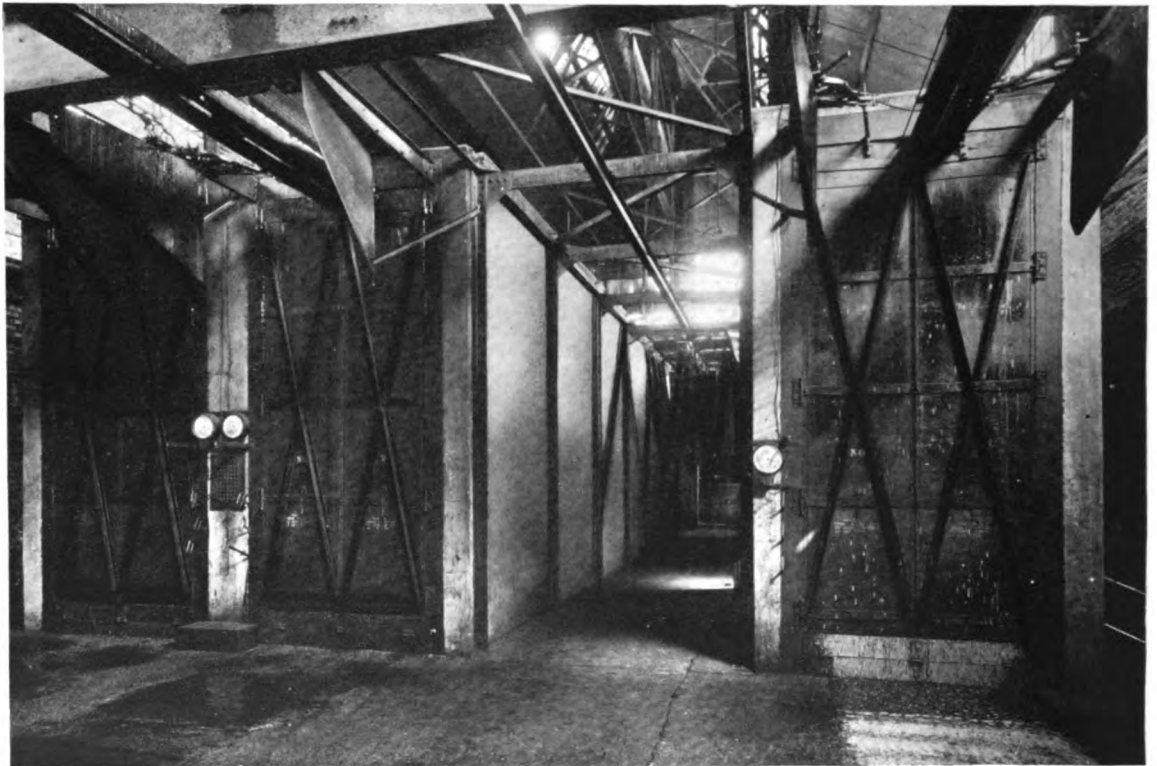
Japanning ovens at the Durand Steel Locker Co., Chicago Heights, Ill., built entirely of Sil-O-Cel C-3 Concrete, 9" thick in walls and tops
