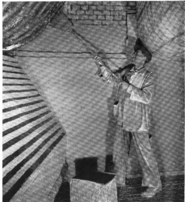
Wash-coating with J-M Refractory Cement
