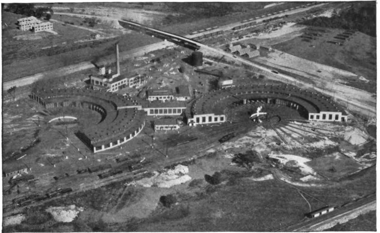
New York Central engine terminal at Selkirk, N. Y., where sixty-five type "N" Moulded Ventilating Transite Smoke Jacks are in service
