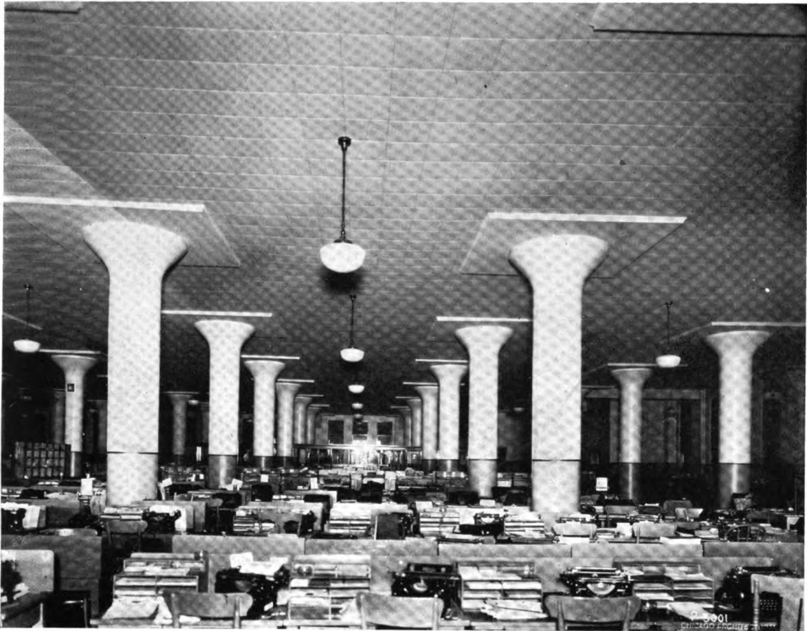
A business office of Montgomery Ward & Co., with Sanacoustic Tile on the ceiling. Progressive organizations are quick to realize that noise control methods constitute a highly profitable investment
