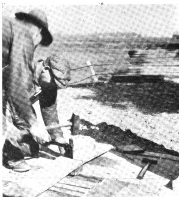
Cutting a J-M Asphalt Bridge Plank
