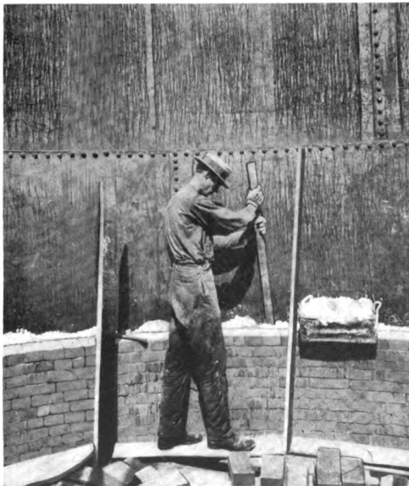
Installing Sil-O-Cel Coarse Grade in wall of vertical lime kiln
