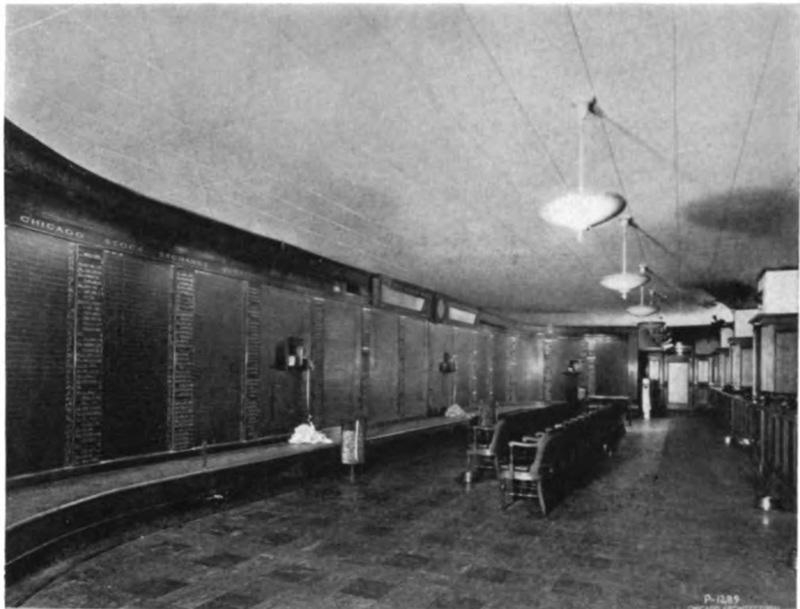
A brokerage office customers' room is the scene of many distractions, but the disturbing effect of noise is probably the worst. Sanacoustic Tile on the ceiling absorbs objectionable sound
