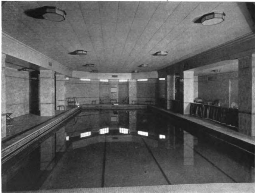
Unless ceilings are treated to absorb sound, the noise of splash and chatter in a swimming pool soon reaches disagreeable proportions, and also endangers the lives of poor swimmers, whose calls for help could pass unnoticed. Sanacoustic Tile and fittings are made of aluminum where dampness is to be encountered
