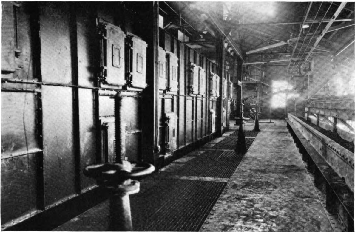
Cottrells insulated on sides with 3" Sil-O-Cel Coarse Grade. Tops are insulated with 2½" of Sil-O-Cel Natural Brick
