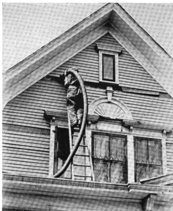
Blowing J-M Home Insulation into the walls of a frame house
