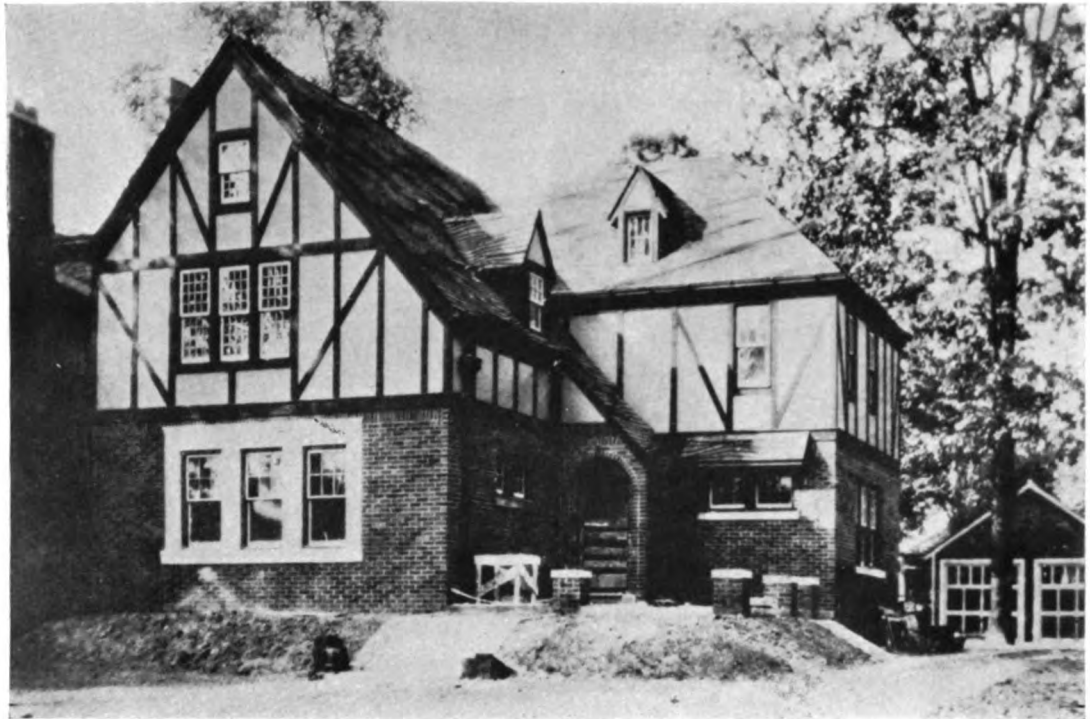
Flat Transite half-timber effects on residence in Detroit, Mich.
