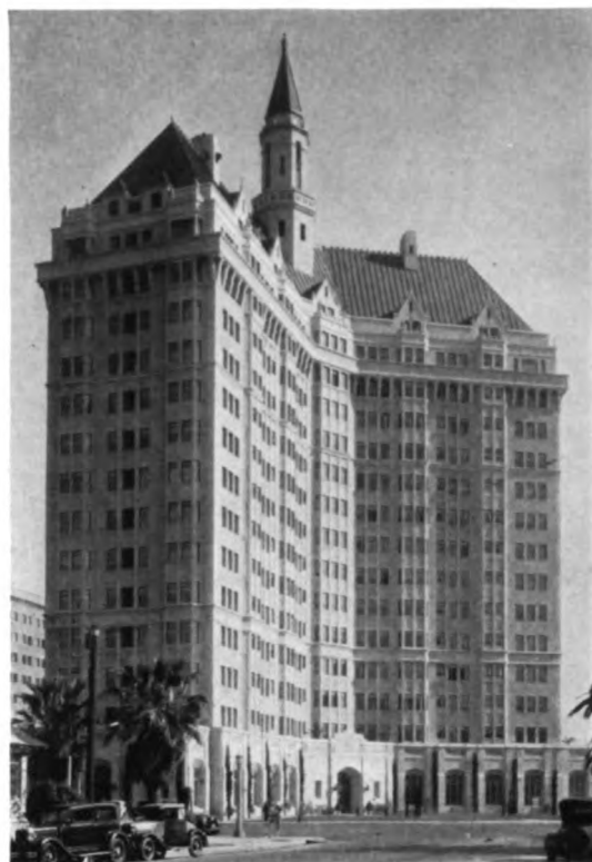
Fig. 6. Villa Riviera, Long Beach, California. Celite proved highly satisfactory in the stucco mixtures used in the construction of this large cöoperatively-owned apartment. Richard D. King, Los Angeles, California, Architect; Kinne & Westerhouse, Los Angeles, California, Contractors
