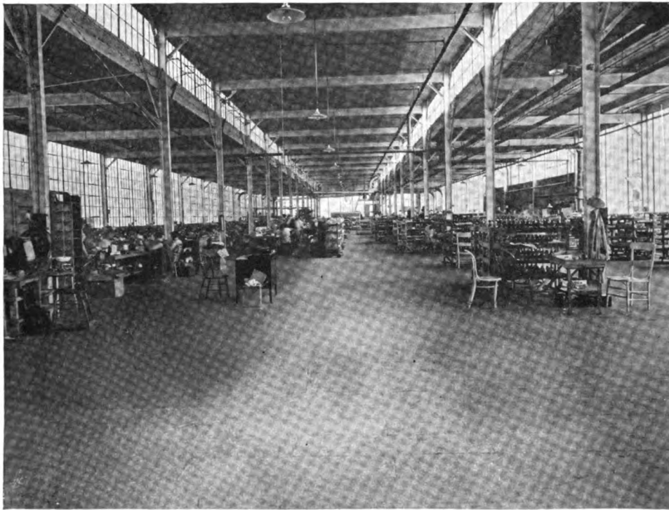
25,000 sq. ft. of 1/2" Industrial Flooring Plank No. 45 at the Stern-Auer Shoe Co., Chillicothe, Ohio, have stood up under chairs and small-castored hand trucks for over a year—and remain as smooth as when laid
