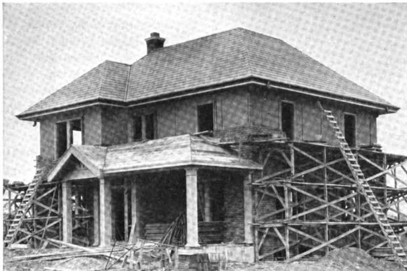
J-M Insulating Board as sheathing under brick veneer
