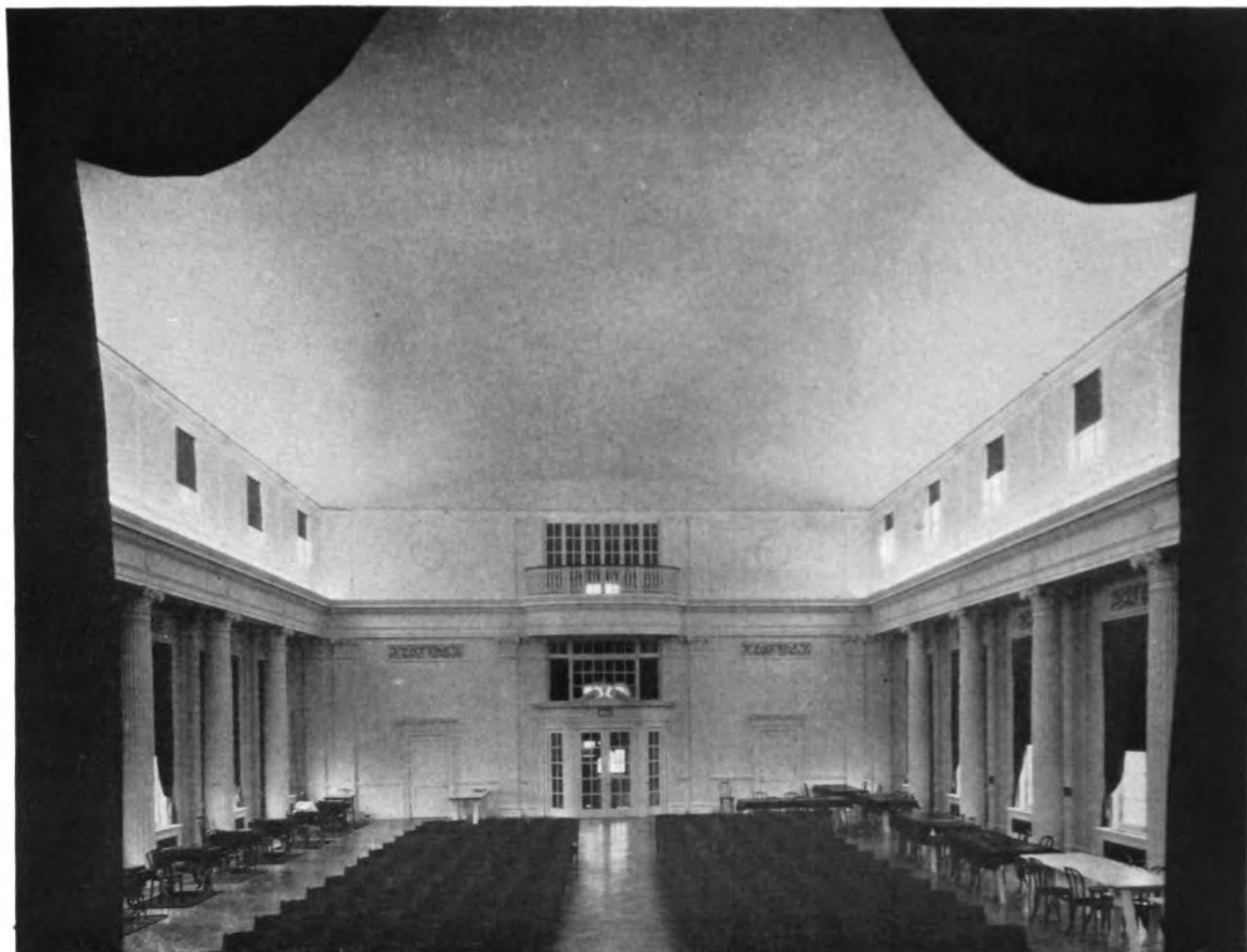
Auditorium in the Women of the World War Building, Washington, D. C., acoustically treated with Nashkote Type B
