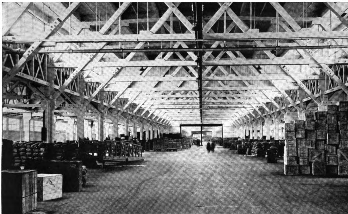
J-M Industrial Flooring on Pier B of the Canadian Pacific Ry. at Vancouver, B. C.
