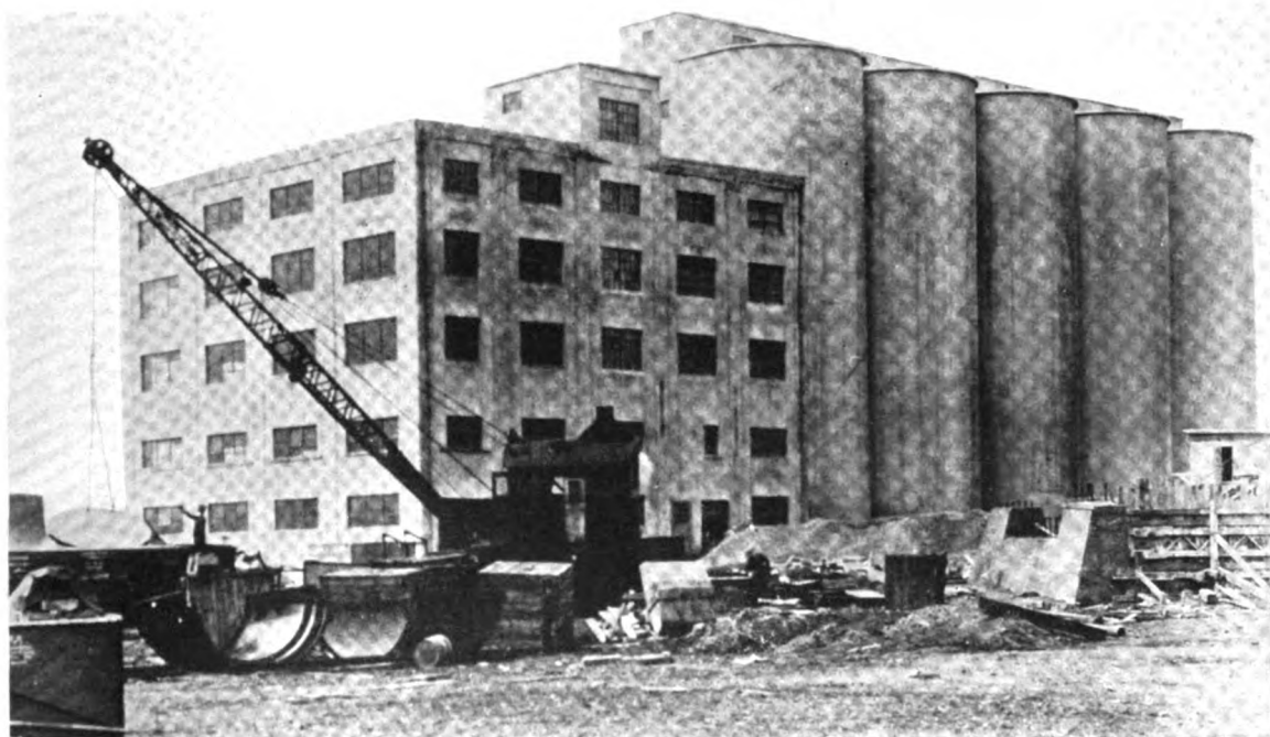
Fig. 9. Keystone Portland Cement Company, Bath, Pennsylvania. 4 lb. (0.4 cu. ft.) of Celite per bag of cement in a 1:2:4 mix slag aggregate. R. K. Mead, Baltimore, Maryland, Consulting Engineer; M. A. Long, Baltimore, Maryland, Contractor
