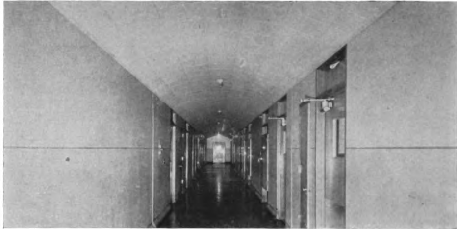
Corridor in Billings Memorial Hospital, University of Chicago, treated with Sanacoustic Tile
