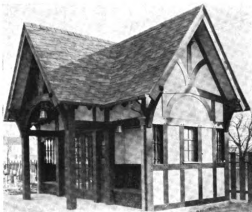
Standard Oil Co. filling station, Cleveland, O., sided with Rough Cast Transite
