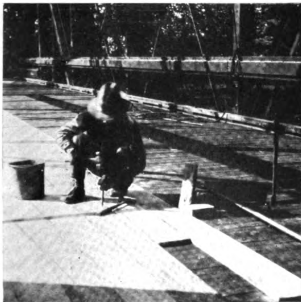
Countersinking nails in J-M Asphalt Bridge Plank
