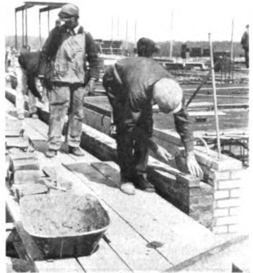
Fig. 2. The use of Celite in brick mortars improves the working properties of the mixture, increases the spread and helps to assure an impermeable joint of neat appearance
