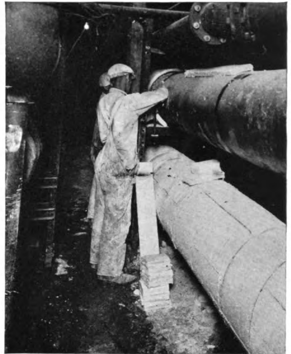
Large steam lines being insulated with J-M 85% Magnesia, Double Standard Thick
