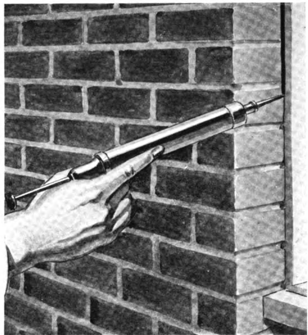
J-M Asbestos Caulking Putty being applied with a caulking gun
