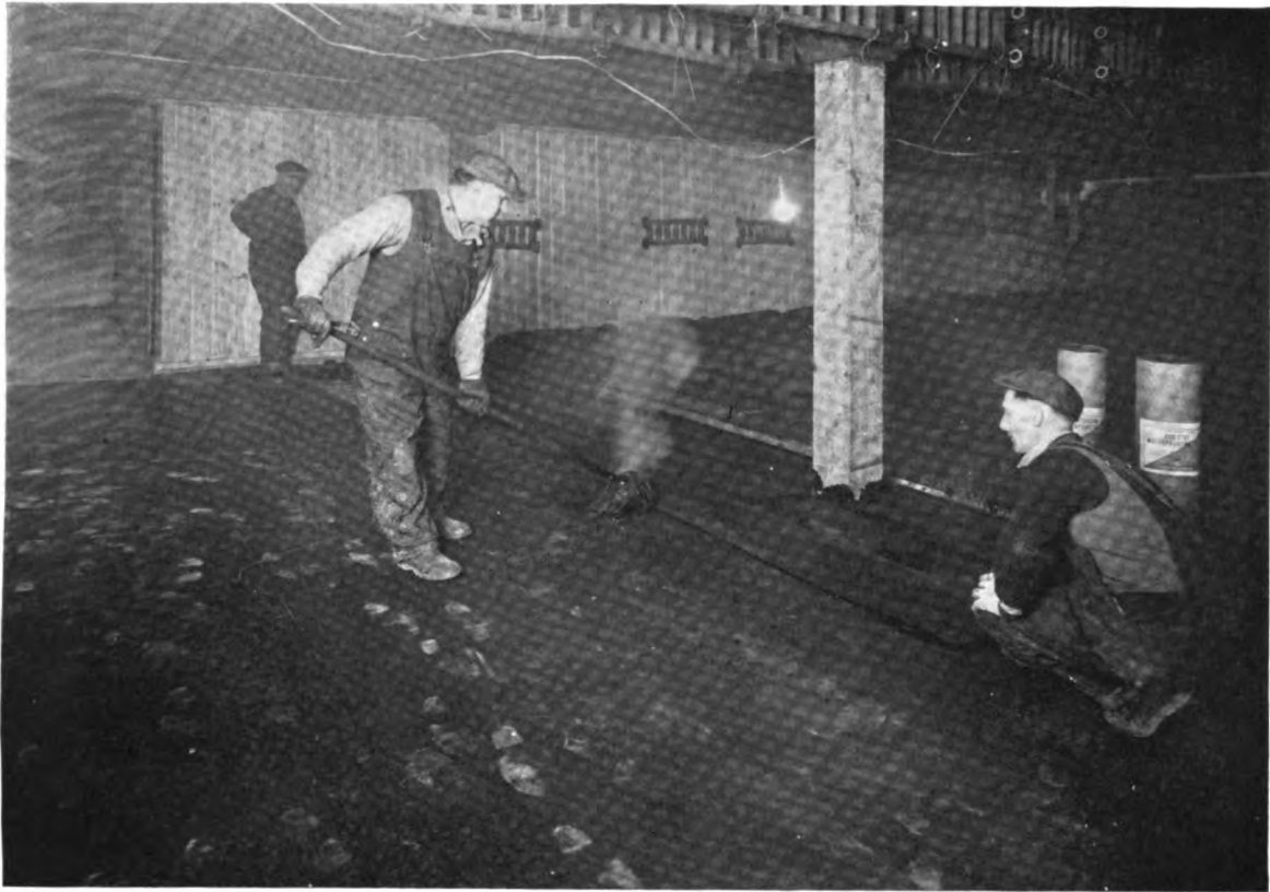
Mopping-in J-M Asbestos Waterproofing Felt
