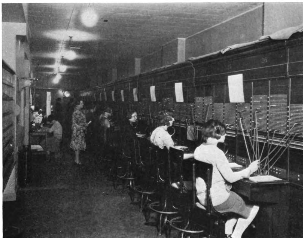
Sound control is indispensable in the telephone exchange. This installation of Sanacoustic Tile is in the Hotel Pennsylvania, New York City
