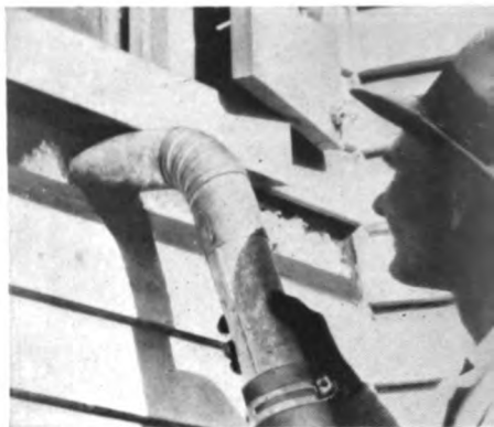
Circle: From a man-made volcano comes rock wool, four inches of which is as effective in insulating the wall of a home as would be eleven feet of solid stone. Above: In existing homes rock wool, in nodulated form, is blown under pressure into hollow walls and attic spaces. Left: For new construction rock wool is applied in the form of batts.
