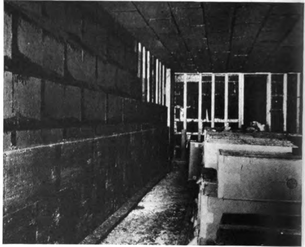
One of more than thirty installations of Rock Cork in New York City plants of the Dairymen's League. The dairy, ice cream and other food products industries have learned to depend upon J-M Rock Cork sheets for efficient, permanent insulation of cold rooms.
