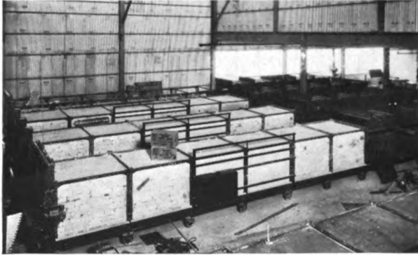
Four electrically heated lehrs for annealing glass, heavily insulated with Sil-O-Cel Super Brick as the inner lining, backed up with Sil-O-Cel Natural Brick. Ten inches of insulation was used in bottom, sides and top.
