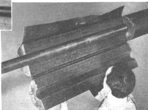
Above: Installing Johns-Manville Rock Cork Sheets. Many such installations are in perfect condition after more than thirty years of service. Right: Applying a section of J-M Rock Cork Pipe Insulation. Note the waterproof jacket with lap for sealing which is an integral part of the pipe covering itself.
