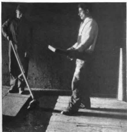
Above: Installing Johns-Manville Rock Cork Sheets. Many such installations are in perfect condition after more than thirty years of service. Right: Applying a section of J-M Rock Cork Pipe Insulation. Note the waterproof jacket with lap for sealing which is an integral part of the pipe covering itself.
