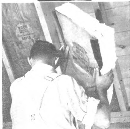
Circle: From a man-made volcano comes rock wool, four inches of which is as effective in insulating the wall of a home as would be eleven feet of solid stone. Above: In existing homes rock wool, in nodulated form, is blown under pressure into hollow walls and attic spaces. Left: For new construction rock wool is applied in the form of batts.
