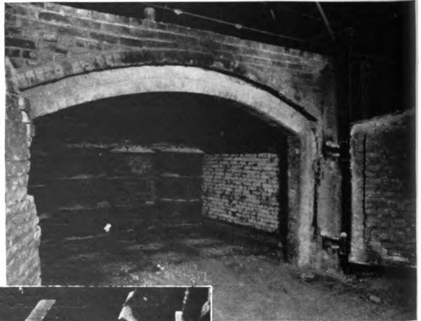
Above: One of six malleable annealing furnaces in the Canton Malleable Iron Company, Canton, Ohio. In these furnaces Sil-O-Cel C-22 Brick is used as a combination insulation and refractory lining for walls, roofs and doors. For the past six years C-22 Brick has saved enough fuel to pay over 100 per cent annual return on its cost, and is still in perfect condition. Left: Here Sil-O-Cel C-22 Brick is used in "core wall" construction behind the fire brick lining in the furnace wall of an oil-cracking unit.
