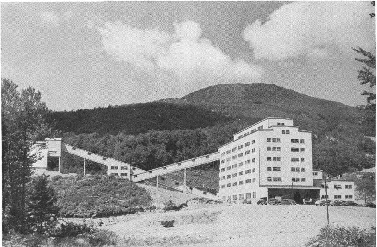
FIGURE 4.—Mill of Vermont Asbestos Mines, Near Eden, Vt.
