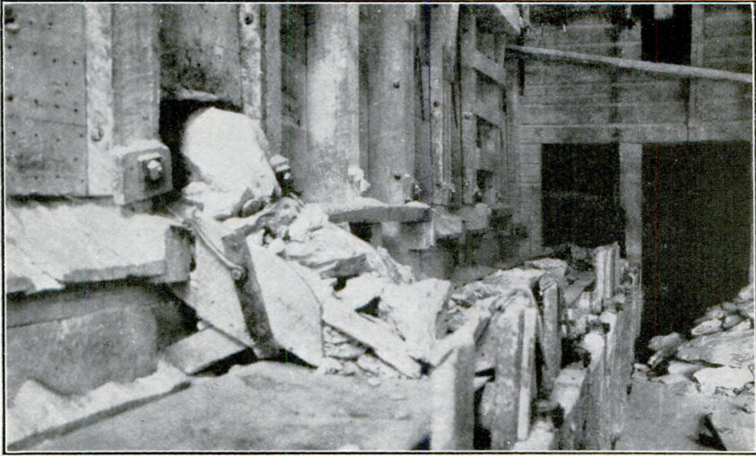
A. FEED SPOUT FOR BELT CONVEYOR. MAGNESIA TALC CO., WATERBURY, VT.
