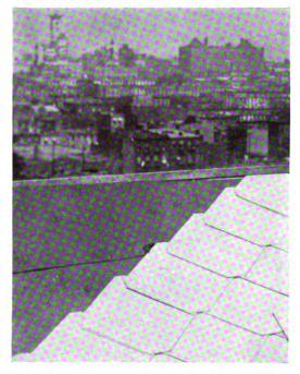
Asbestos Slater's Felt as a liner under Asbestos Shingles
