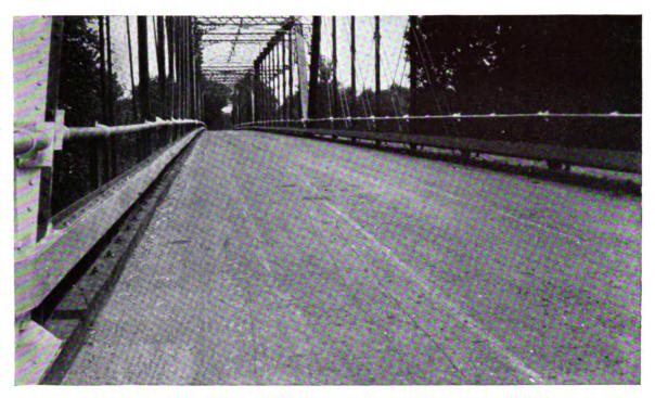
J-M Asphalt Plank on bridge for Ohio State Highway Department, Circleville, Ohio
