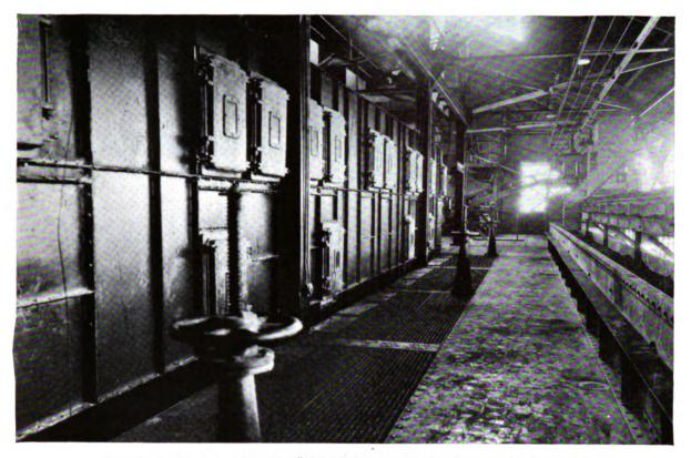
Cottrells insulated on sides with 3" Sil-O-Cel Coarse Grade. Tops are insulated with  $2\frac{1}{2}$ " of Sil-O-Cel Natural Brick
