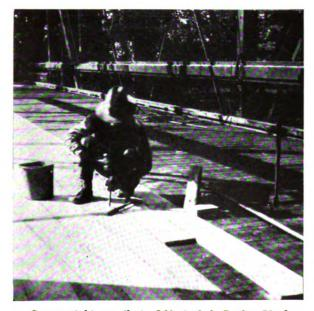
Countersinking nails in J-M Asphalt Bridge Plank
