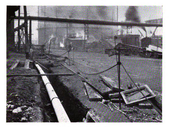
Twelve-inch Class B Transite Pipe for water mains in a large gas plant
