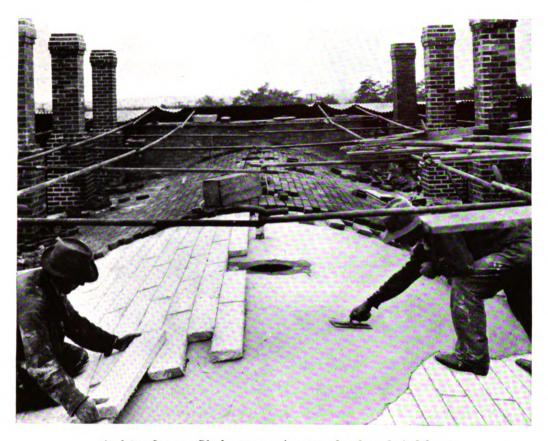
Applying Superex Blocks to top of rectangular down-draft kiln at Hazelton Brick Co., Hazelton, Pa.
