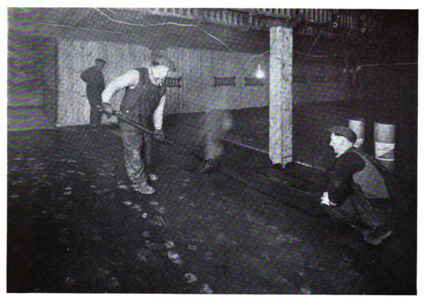
Mopping-in J-M Asbestos Waterproofing Felt
