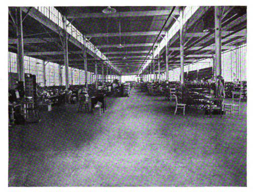
25,000 sq. ft. of <sup>1</sup>/<sub>2</sub>" Industrial Flooring Plank No. 45 at the Stern-Auer Shoe Co., Chillicothe, Ohio, have stood up under chairs and small-castored hand trucks for over a year—and remain as smooth as when laid
