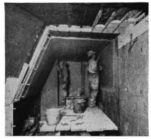
Boiler breeching lined with 2½" Sil-O-Cel Natural Brick and Semi-Refractory Cement
