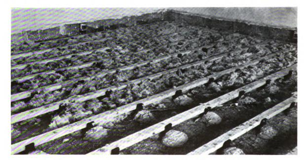
In fireproof apartment sound-isolation construction, J-M floor chairs are grouted in with cement. Sound isolation fill is placed between the stringers
