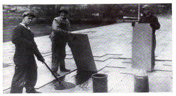
Three layers of  $\frac{1}{2}$ " J-M Rigid Roofinsul, to be overlaid with a J-M Built-up Roof
