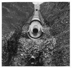
In the J-M System the conduit is completely filled with asbestos fibre, and adequate drainage provided by bell and spigot pipe in broken stone
