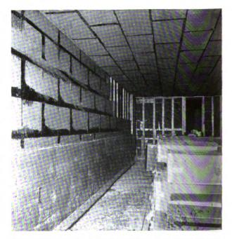
In building solid Rock Cork partitions as at the left and in the background, the first layer is stuck to the temporary studding and the second layer applied in a  $\frac{1}{2}$ " bed of portland cement mortar
