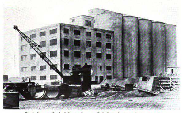
Fig. 9. Keystone Portland Cement Company, Bath, Pennsylvania. 4 lb. (0.4 cu. ft.) of Celite per bag of cement in a 1:2:4 mix slag aggregate. R. K. Mead, Baltimore, Maryland, Consulting Engineer; M. A. Long, Baltimore, Maryland, Contractor
