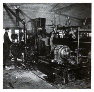
Mechanical spiral wrapping machine for mill wrapping. Applying the asbestos felt to the bitumen-coated pipe
