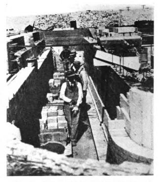
Underground flue insulated with two  $1\frac{1}{2}$ " layers of Superex between 9" of fire brick and concrete outer wall
