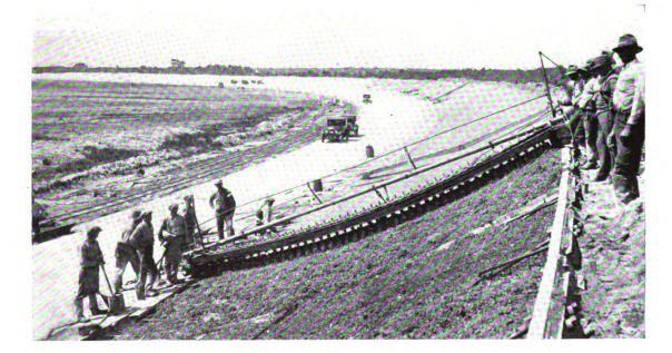
Fig. 3. Test track—2.5 miles long—of Packard Motor Car Co., near Utica, Michigan. 2 lb. or 0.2 cu. ft. Celite per bag of cement gave excellent results, enabling "dry" mix to be used, and giving perfect finish. Uniformity secured with Celite insures full effective slab thickness. R. D. Baker Co., Contractors
