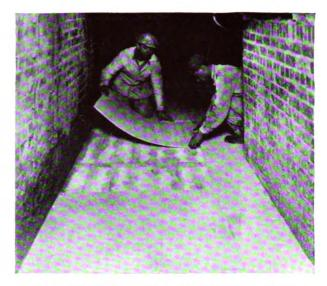
Laying J-M Millboard over Superex blocks between side walls and brick pier in base of asphalt still
