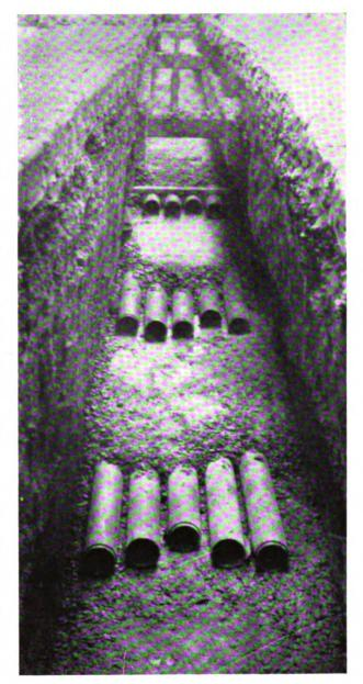
Orangeburg Fibre Conduit laid tier-by-tier method in a 14-tube bank
