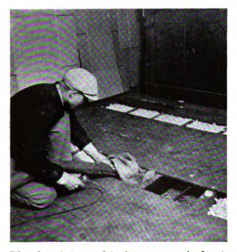
When the attic is unused for living quarters, the floor is insulated to stop heat leakage through the rooj
