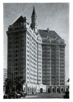
Fig. 6. Villa Riviera, Long Beach, California. Celite proved highly satisfactory in the stucco mixtures used in the construction of this large cöoperatively-owned apartment.
