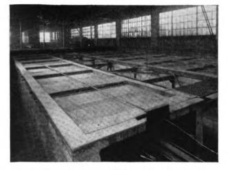
Large japanning ovens at the Durand Steel Locker Co., Chicago Heights, Ill., built entirely of Sil-O-Cel C-3 Concrete with 9" thick walls and tops. Size of ovens 9 ft. wide, 22 ft. high, 50 ft. long
