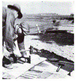
Cutting a J-M Asphalt Bridge Plank
