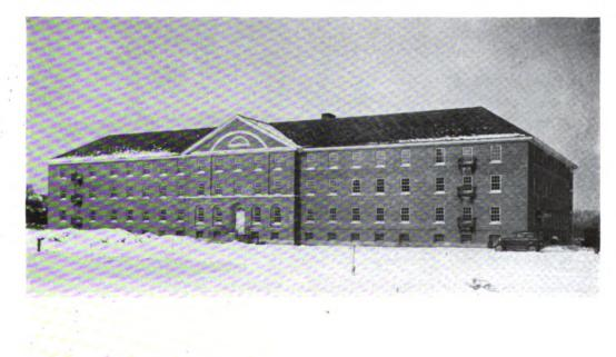
Fig. 3. Nurses House, Department of Mental Diseases of Commonwealth of Massachusetts, Waltham, Mass. Celite was used in all mortars in proportions varying from 0.6 to 0.8 cu. ft. (6 to 8 lb.) per bag of cement. Gordon Robb, Boston, Architect; Cummings, Matthews Co., and C. S. Cunningham & Sons Co., Boston, Contractors
