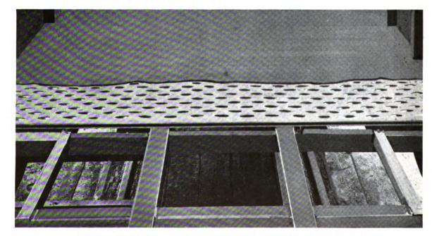
J-M Truss Plate bolted to car beams and overlaid with J M Masticoke Flooring
