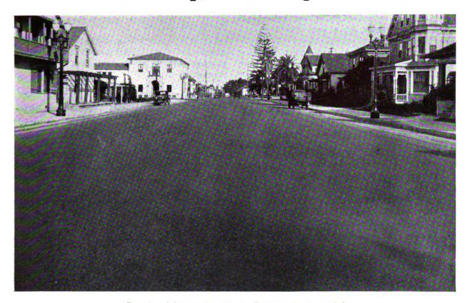
Fig. 1. Celite used with excellent results in asphalt paving on Chapala Street, Santa Barbara, Calif. Richardson Construction Co., Santa Barbara, Calif., Contractors
