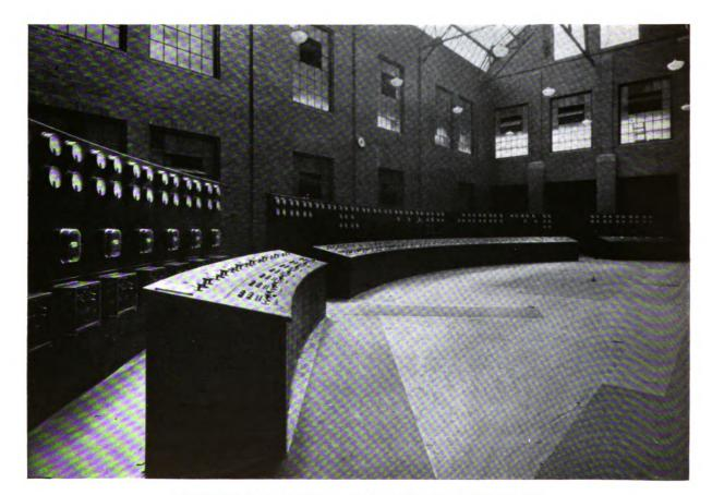
North Side Pumping Station, Sanitary District of Chicago, Ill. Control bench and instrument boards of Asbestos Ebony
