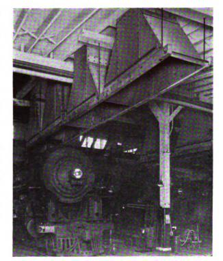
New York Central engine terminal at Harmon, N. Y., showing four Transite Smoke Jacks in tandem over the drop pits
