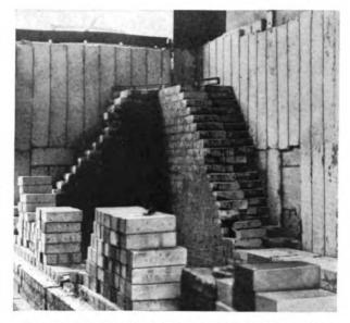
Superex Combination Insulation,  $3\frac{1}{2}$ " thick, between Transite casing and fire brick lining of Gyro tube still
