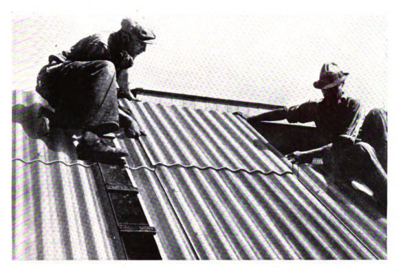
Laying J-M Corrugated Transite Roofing. The cut corner construction permits a tight joint with straight lap lines, and results in a durable, attractive roof
