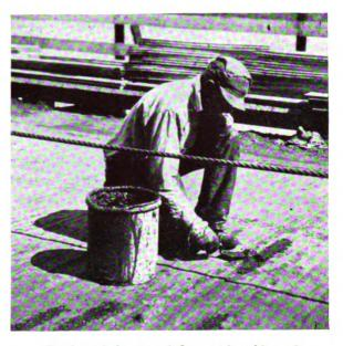
Patching holes in sub-floor with cold patch material before laying Asphalt Bridge Plank
