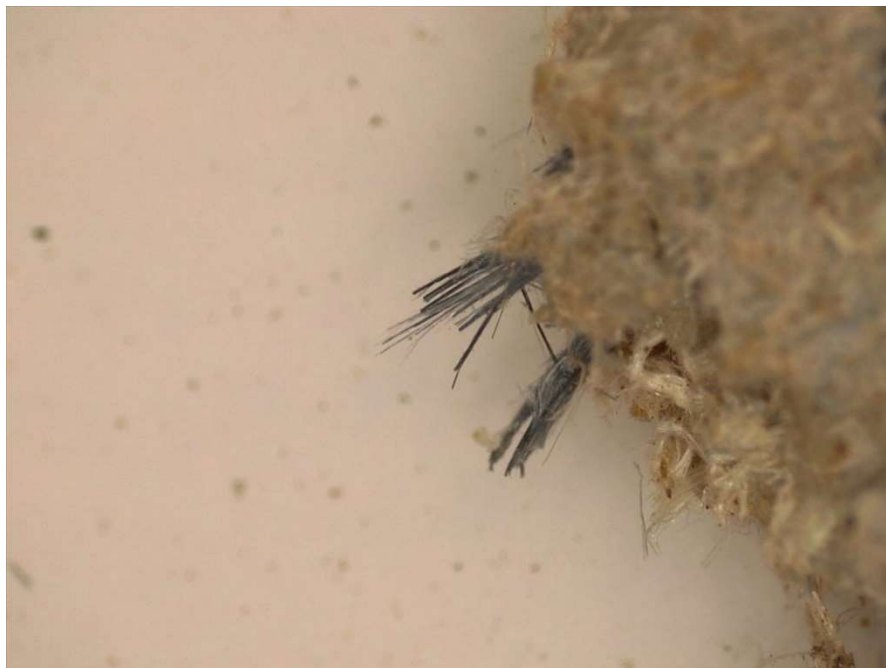
Crocidolite (Blue Asbestos) Fibers being Liberated to the Environment from a Deteriorating Asbestos-Cement Pipe Picture Courtesy of Joe Frasca
